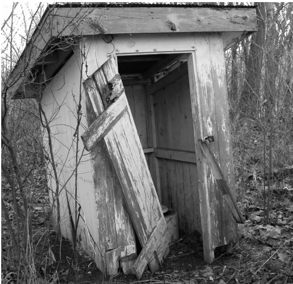
This outhouse sat for years in Six Crossings Hollow near Duke until the Big Piney flushed it downstream in the flood of 2008.
