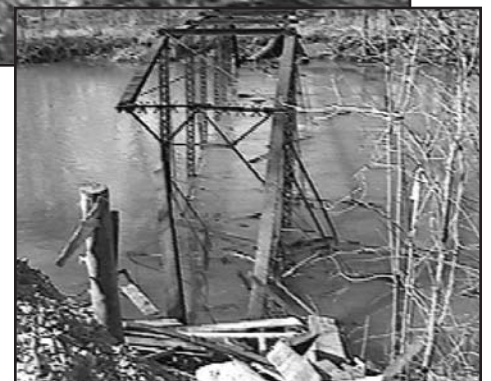
In the montage above, an Army demolition expert (top) ties on plastic explosives. Center, the bridge is engulfed in red/yellow flame (bright white in the b/w photo.) Lower right, the superstructure has been blown off its piers and sits on the river bottom.
