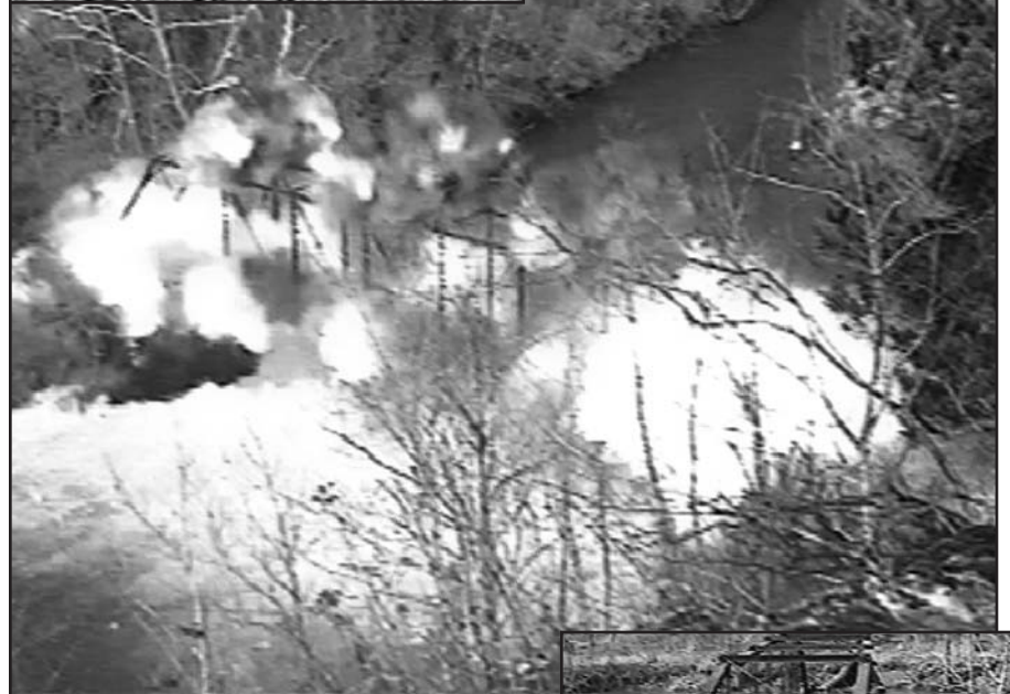
In the montage above, an Army demolition expert (top) ties on plastic explosives. Center, the bridge is engulfed in red/yellow flame (bright white in the b/w photo.) Lower right, the superstructure has been blown off its piers and sits on the river bottom.
