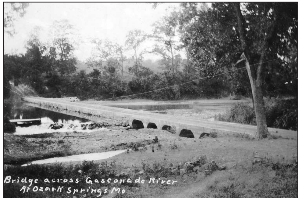
The county also has a number of low water bridges, mostly unnamed, such as this one at Mays Ford at Ozark Springs resort. It is of more recent construction than the others pictured on these pages. Courtesy of John Bradbury.
