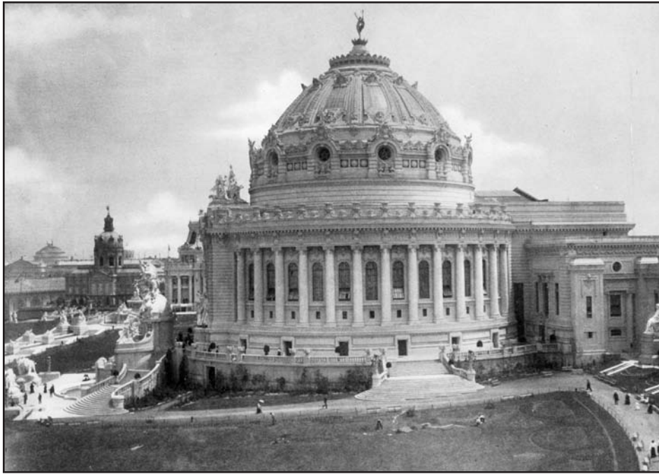
Festival Hall was the greatest auditorium on the World's Fair grounds. The dome was one hundred and sixty-five feet in diameter and one hundred and ninety feet tall, exceeding that of St. Peter's. The auditorium seated over three thousand people and housed the largest pipe organ ever built.
