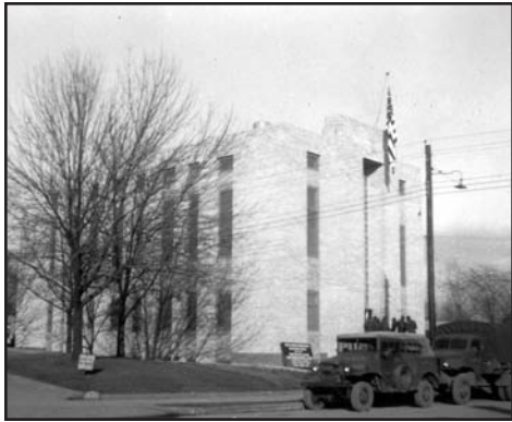
Although a little smaller, a similarly designed Colored USO Club was constructed in Rolla. It now serves as part of the City Hall complex. Courtesy of the Mann Collection, Western Historical Manuscript Collection, University of Missouri-Rolla.
