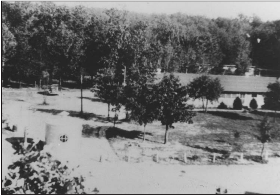
This is a view along the main road of the camp. The large building in the background is the Forest Service Quarters. The Forest Service and the Army operated the CCC camps. Courtesy of Western Historical Manuscript Collection—Rolla.
