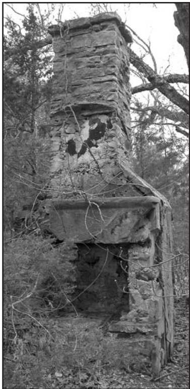
The native stone chimney of the Recreation Hall still stands amid the foundations and rock work at the isolated site of Blooming Rose. Photo by Terry Primas.
