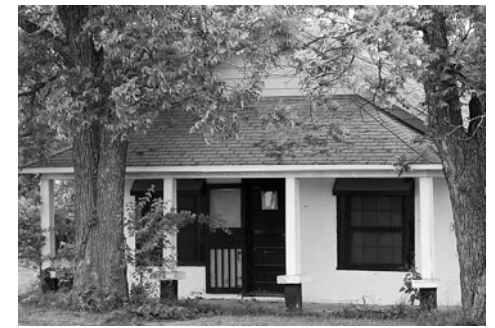
The lone building from Bloodland left standing. Herb and Leora Chambers lived in this house when Herb worked the cows.
