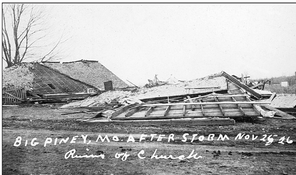
Organized in 1869 on the east side of the Big Piney River, the Hopewell Church congregation built a new church in Big Piney in 1896. The frame building was hit on Thanksgiving Day in 1926 by a tornado (see panorama of the town destruction on page 52). Courtesy of John Bradbury.
