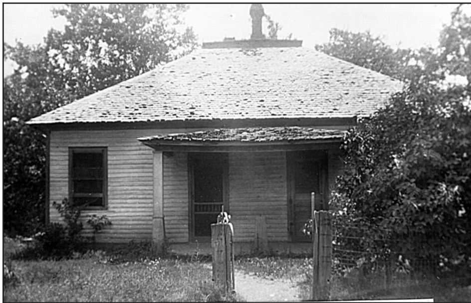
The small house at one of the jogs in the road, denoted as “Eliza’s (Hicks) House” on the map on the preceding page.
