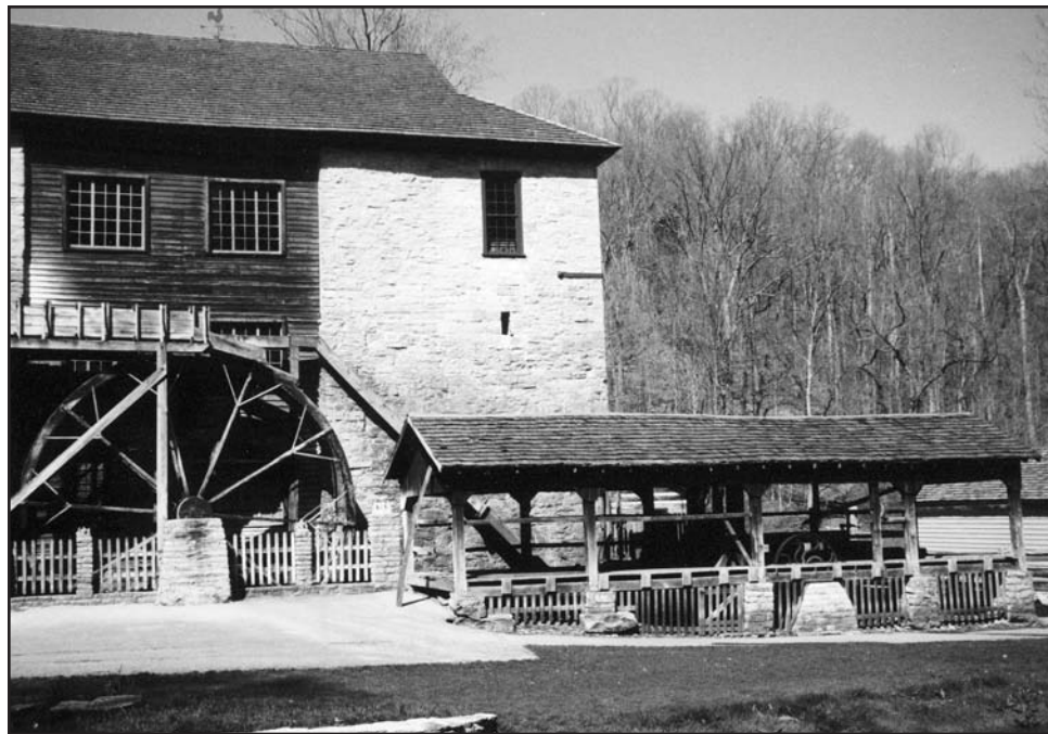
The sash mill was a low slung structure with open sides. A flume diverted water from a nearby spring or watercourse to turn the wheel that powered the up-and-down saw blade. Pictured is one of the few operational water-powered sash mills in the country at Spring Mill State Park near Mitchell, IN. Photo by John Bradbury.
